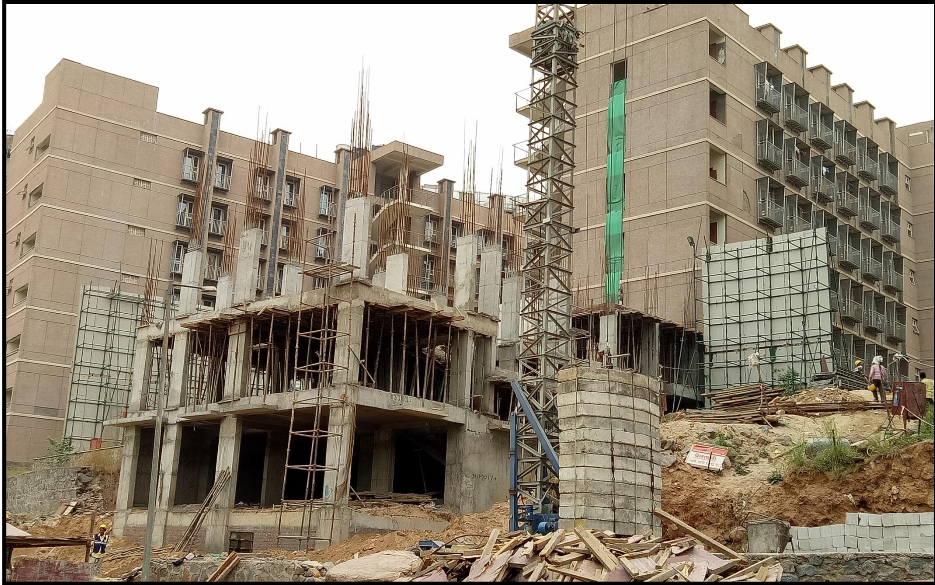
Extension Hostel Blocks B1
