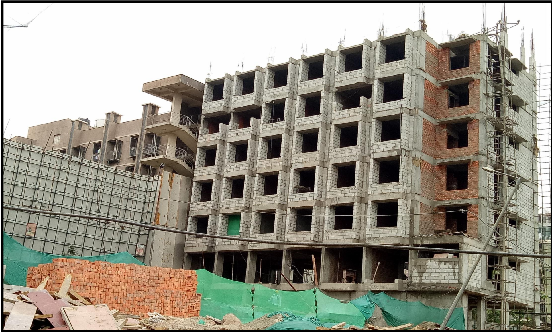
Extension Hostel Blocks G1
