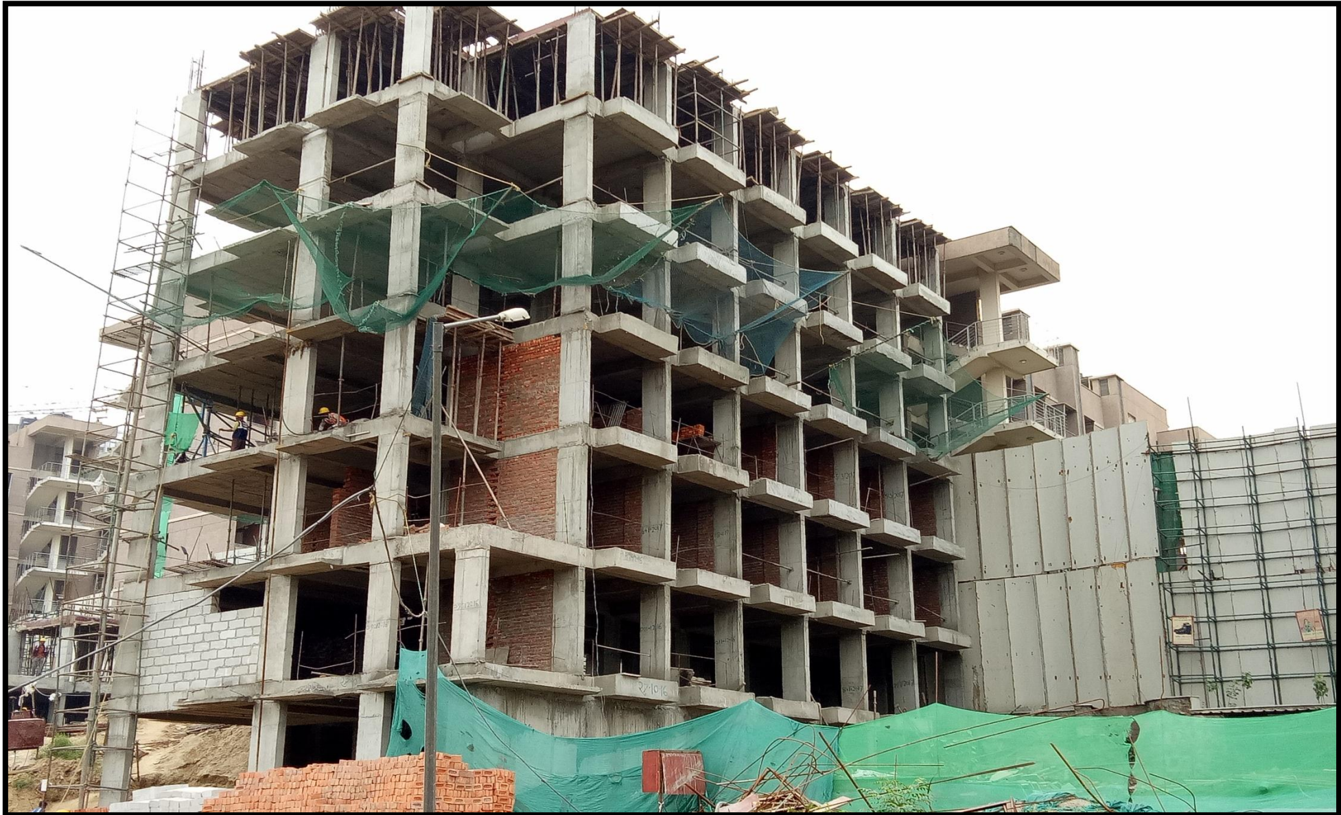
Extension Hostel Blocks G2
